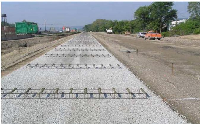
Dowels on steel basket before concrete layout, Turgeon and al. (2009)
